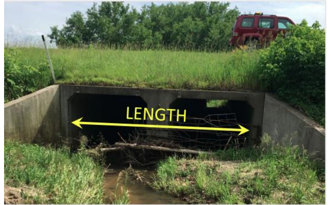
Double Barrel (multicell) Box Culvert
