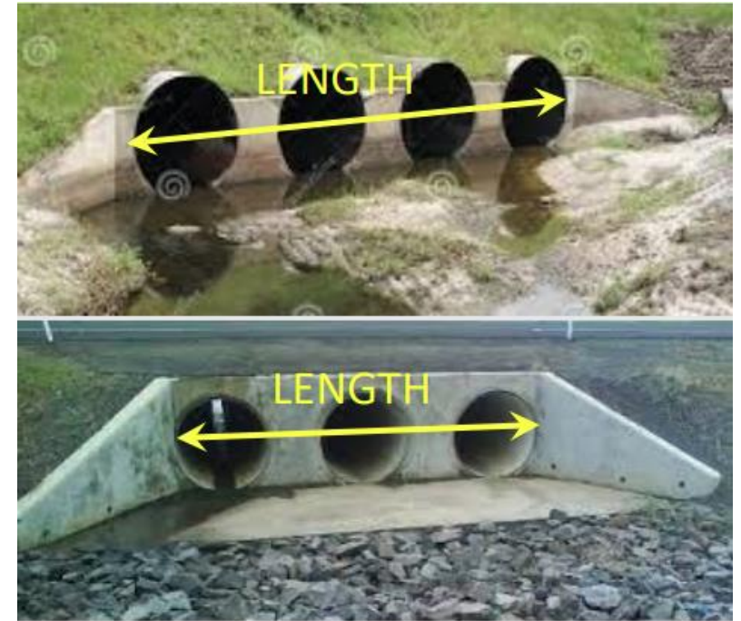
Multiple Pipe Culvert Or “Culvert Nest”
