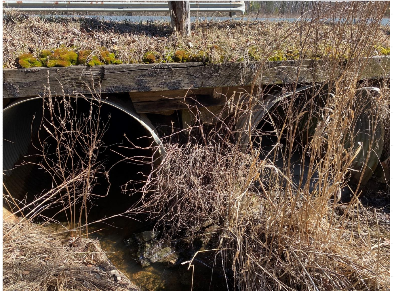
Town of Rudolph – Twin 60" metal culverts to be replaced with 60" plastic
