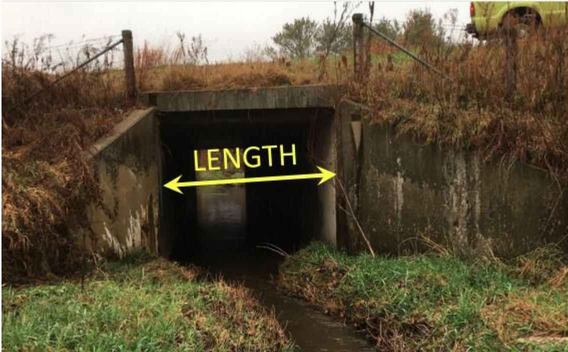
Single Concrete Box Culvert Pipe
